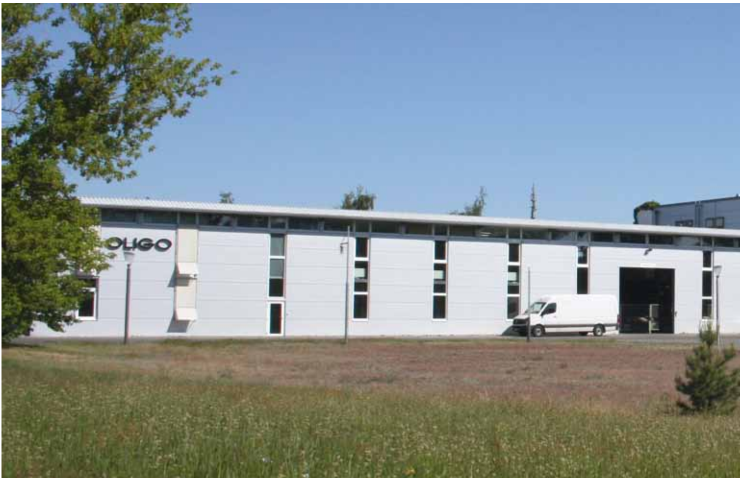
Fig.: Headquarter in Lenzen, Brandenburg
